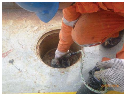
Installed Scupper plugs
