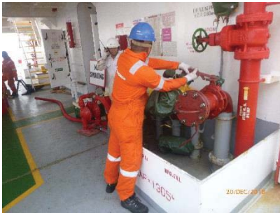
Reporting from bunker manifold
